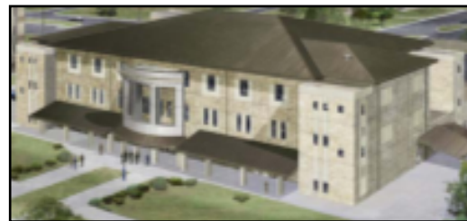
Typical BMT Classroom/Dining Facility JBSA-Lackland
