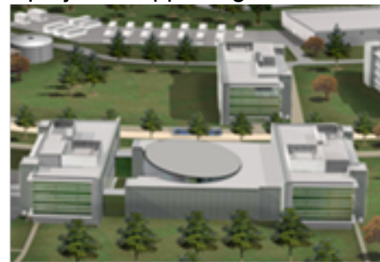
USCYBERCOM Joint Ops Center Ft Meade
